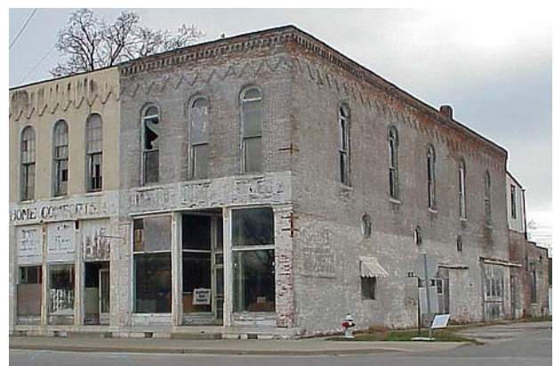
Image 1: Vacant homes and property often become neglected, lowering neighbouring property values.
